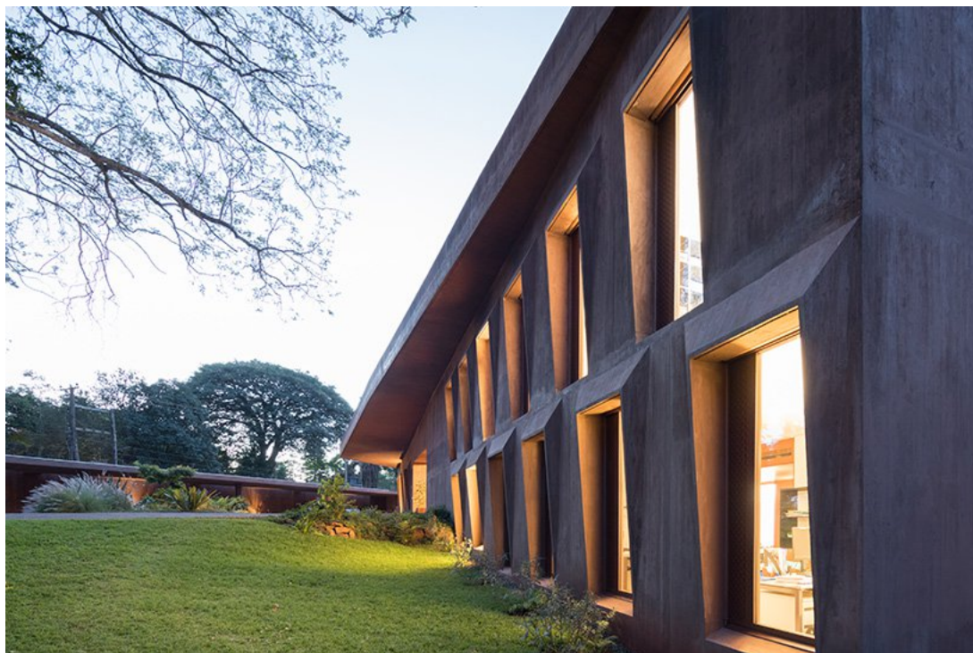
the structure is topped with a green roof image © iwan baan ( https://iwan.com/ )
