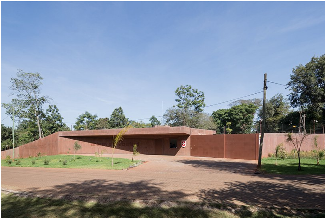
the perimeter wall turned out to be the starting point of the embassy's design image © iwan baan ( https://iwan.com/ )
