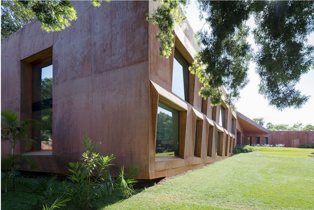
the thick concrete façade regulates the building's internal temperature image © iwan baan ( https://iwan.com/ )
